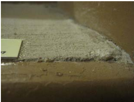
Rising Concrete right before side wall
