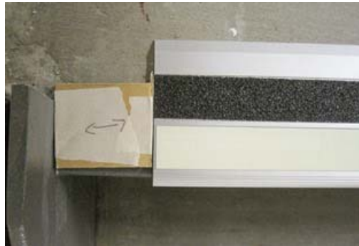
A Space Holder helps maintain exact distance
