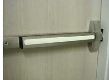
Press Tape onto activating portion of Push Bar. Use a Pressure Roller to apply firm and even pressure over entire length of Tape, therefore squeezing out any air bubbles and making sure the Tape adhesive makes full contact with the Push Bar.
